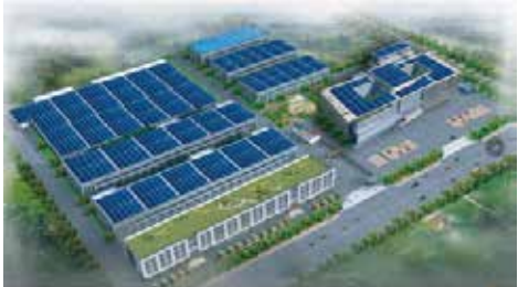
PV&BESS Country :China Configuration : PV 2.85MWp PCS 100KW Battery storage system 460kWh
