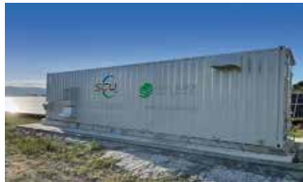
PV&BESS Country : Bulgaria Configuration : PCS 600 KW Battery storage system 1.84MWh
