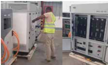
New Energy Charging Station Hybrid storage electric vehicle charging Country : Ethiopia Configuration : GRES-150-150 150kW/150kWh +100kW MPPT
