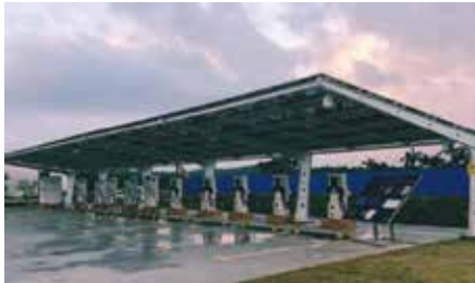
New Energy Charging Station Country :China Configuration : PV 26.68KWp PCS 250KW Battery storage system 550kWh EV charger 300KW
